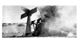
As he was flying the <u>Tallmantz Phoenix P-1</u> over the Arizona desert, the plane struck a small hillock. As Mantz attempted to recover by opening the throttle to its maximum, the over-stressed aircraft broke in two and nosed over into the ground, killing Mantz instantly. <u>https://www.youtube.com/watch?v=n82nN\_lqn58</u> Here's a link to the movie: <u>https://www.youtube.com/watch?v=AxJNxrZCboY</u>
